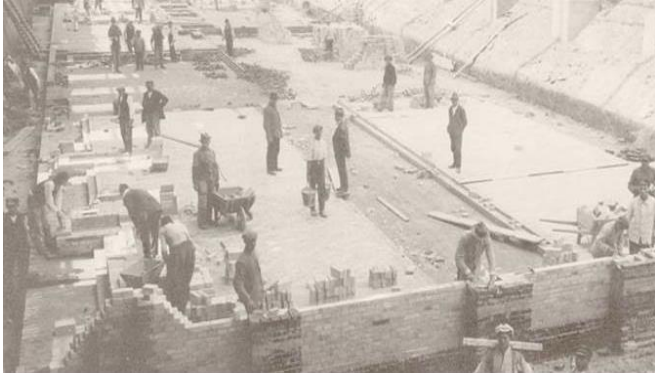
First Riedhammer Baking Furnace
