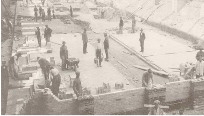
First Riedhammer Baking Furnace
